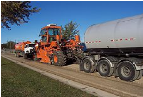
Expanded Asphalt Stabilization
