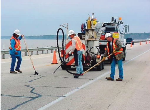
Crack Sealing
