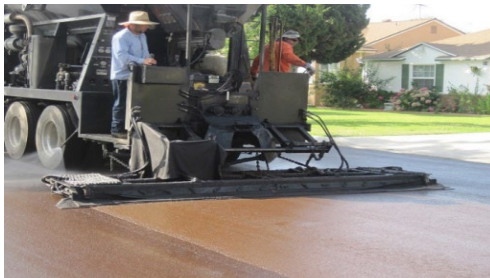
Slurry Seal
