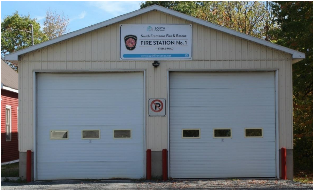
Figure 11. Exterior of Station 1 – Bradshaw.
