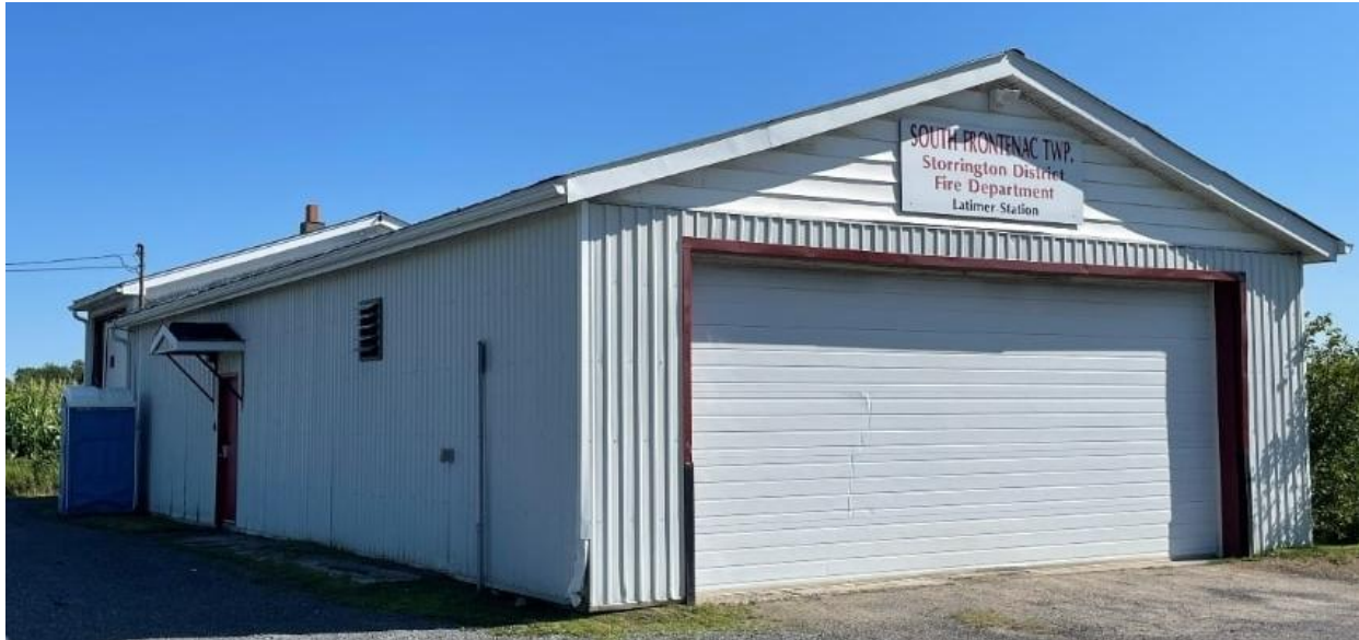
Figure 22. Exterior of Station 7 – Inverary.
