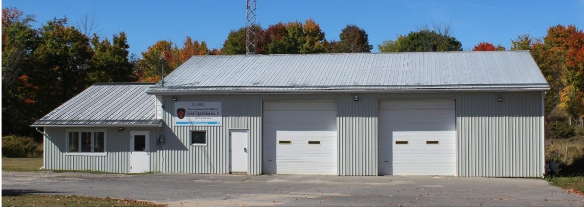
Figure 12. Exterior of Station 2 – Burrige.
