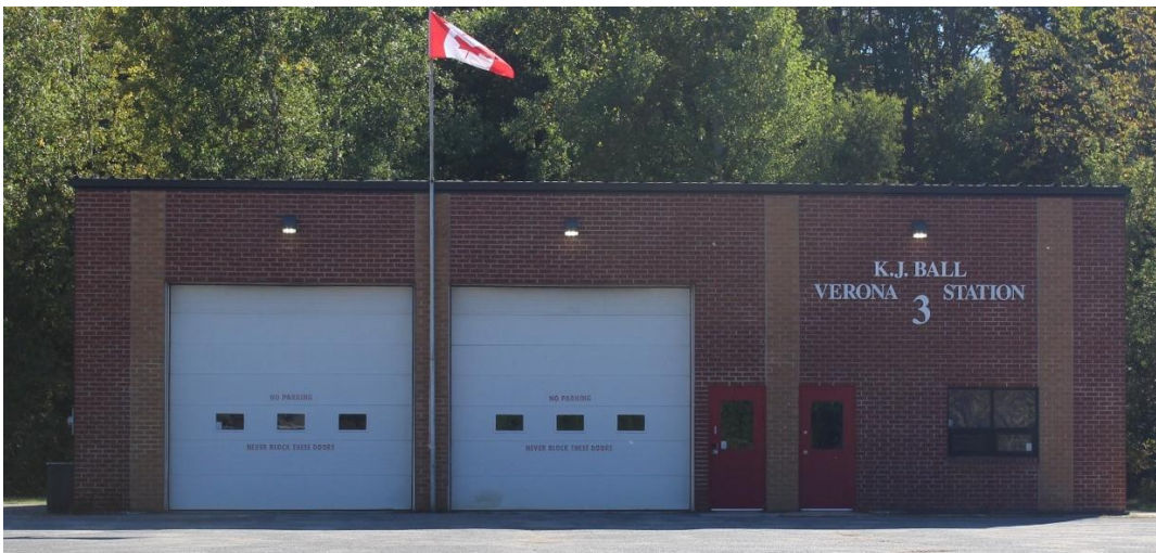
Figure 13. Exterior of Station 3 – Verona.
