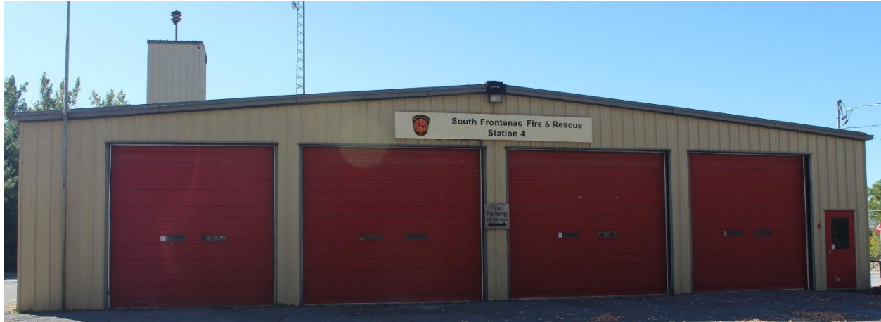
Figure 15. Exterior of Station 4 – Hartington.
