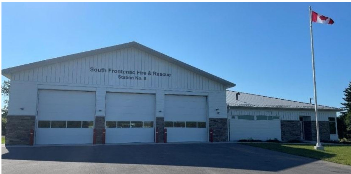
Figure 25. Exterior of Station 8 – Battersea.
