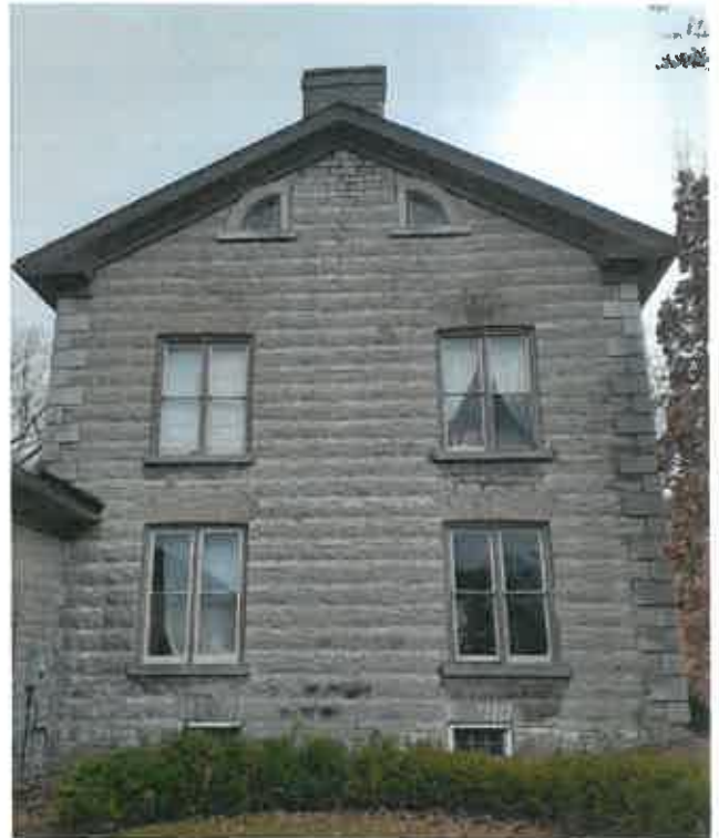
Windows and Attic Storey of Stone House
