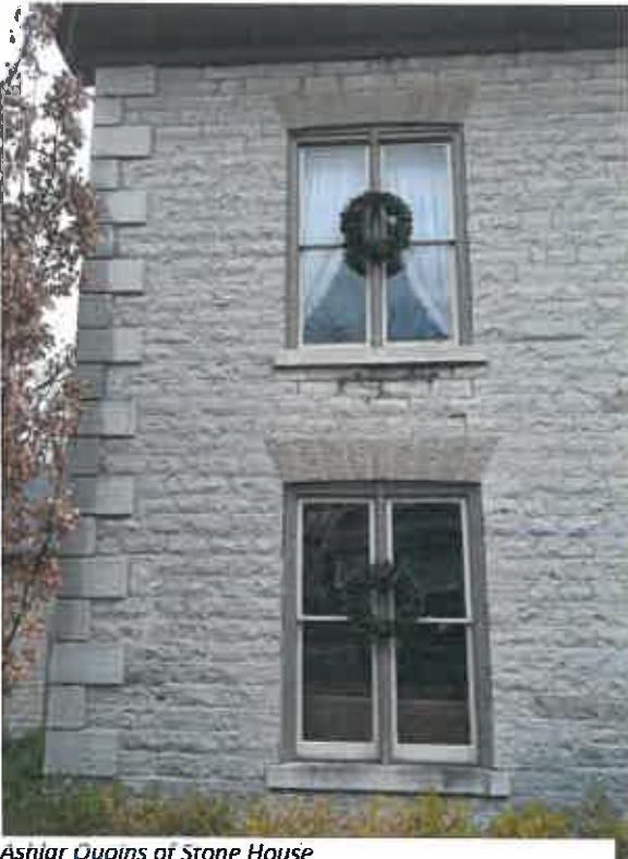
Ashlar Quoins of Stone House
